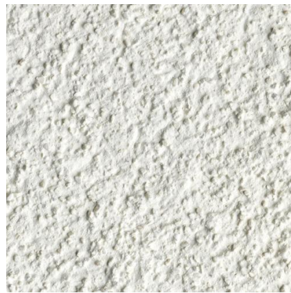
Figure 16: Sand Cement Render Finish
