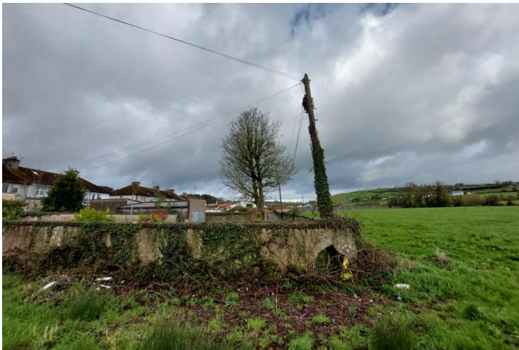
Photo 3: View westwards along existing rear access laneway behind St. Bridget's Villas. Proposed to remove section of wall along new access road to improve the existing laneway access for local residents (to rear of St. Bridget's Villas).
