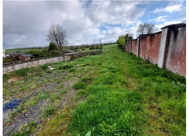
Photo 2: Access road to site (looking north towards the site), existing LHS wall to be removed, existing RHS wall to remain.
