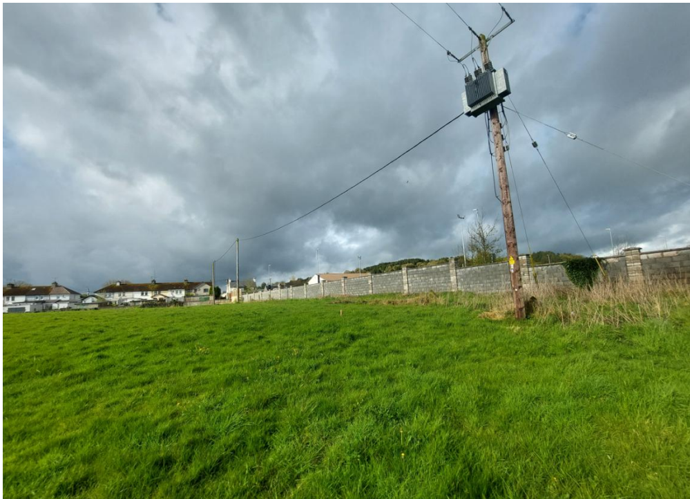
Photo 8: View of existing western boundary wall and existing overhead ESB cables travelling south toward St. Bridet's Villas.
